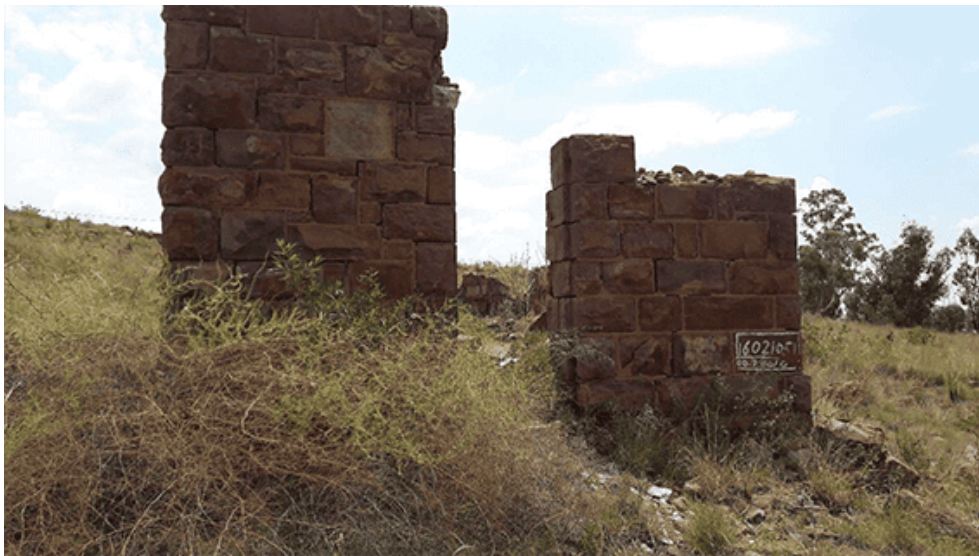
Figure 2: Position of the steel door on the eastern side of the building (Photo: Theo Ligthelm 2017)
