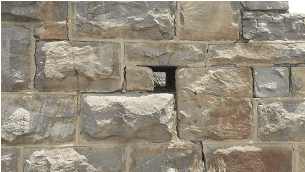
Figure 4: Ventilation holes in walls – (note tunnel design, so these could not have been Loopholes) (Photo: Theo Ligthelm 2017)
