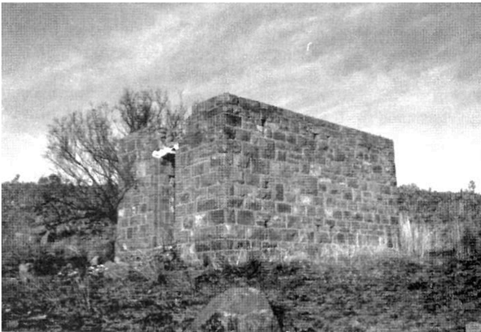
Figure 4: Ventilation holes in walls – (note tunnel design, so these could not have been Loopholes) (Photo: Theo Ligthelm 2017)
