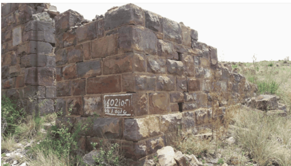
Figure 3: Ventilation holes in the walls – (these have been misinterpreted as loopholes, but have no wider area on the inside, which would therefore make pelleting with a weapon impossible) (Photo: Theo Ligthelm 2017)
